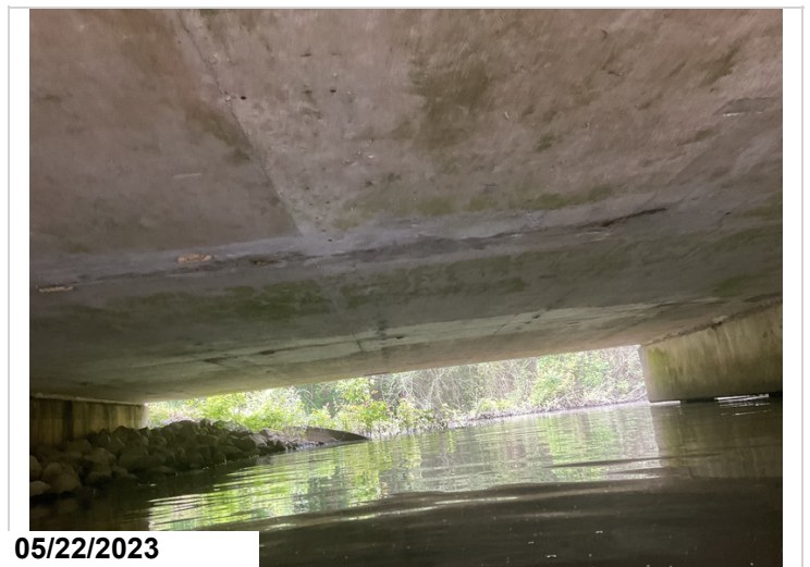
Span 1 soffit has large crack in same location as top of deck. Staining and moisture present.
