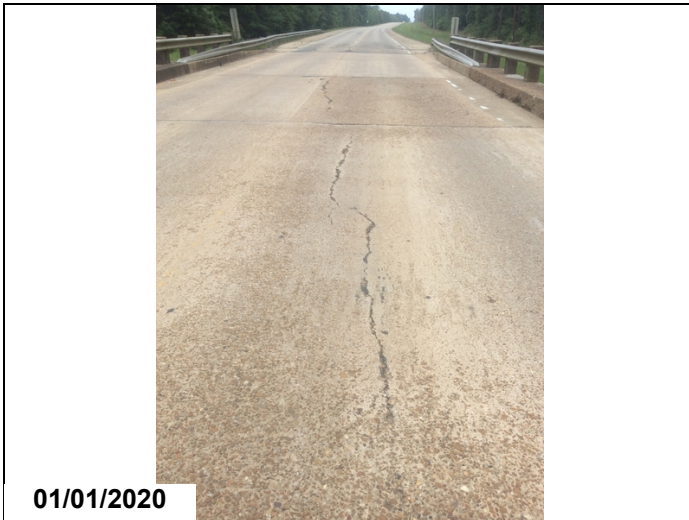
Span 1 Deck cracking
