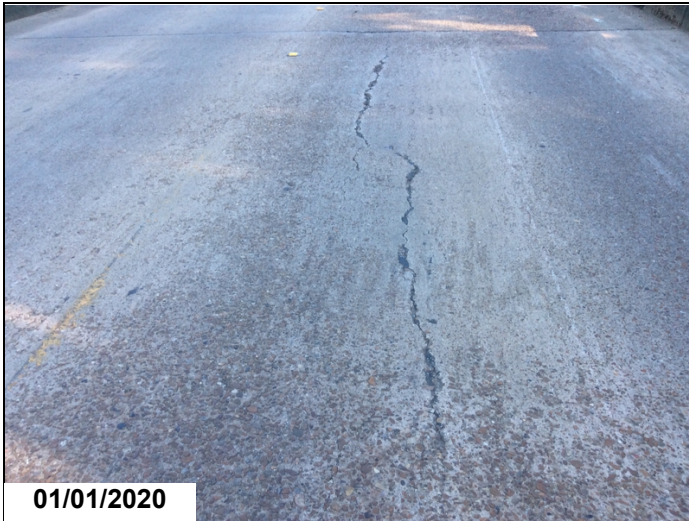
Span 1 Deck cracking
