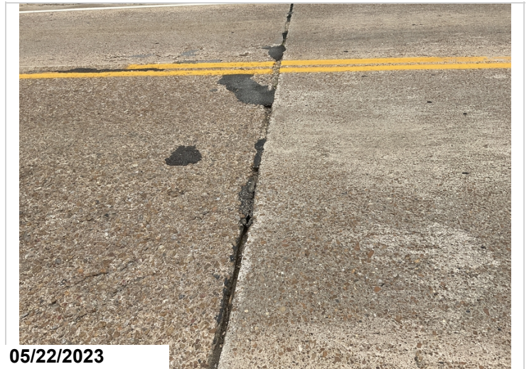
Bent 3 joint seal has lost bond with debris impaction.
