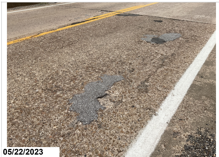
Span 2 deck abrasion with asphalt patches.
