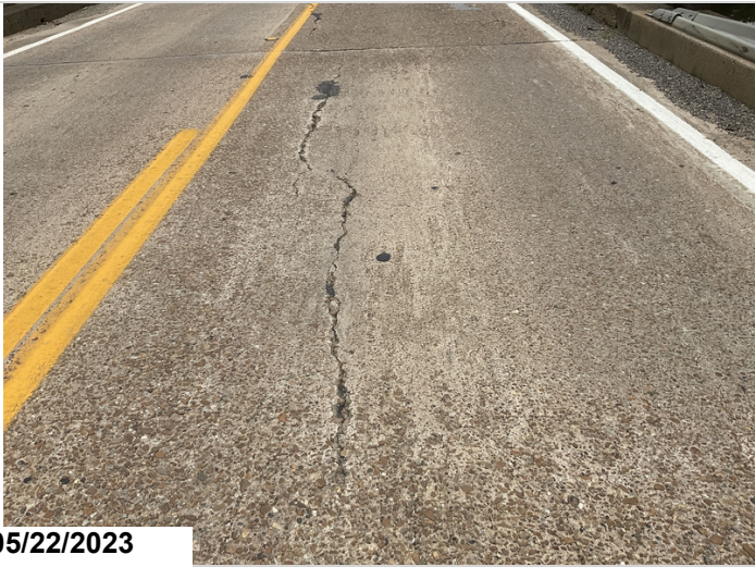
Deck span 1 large unsealed cracks.
