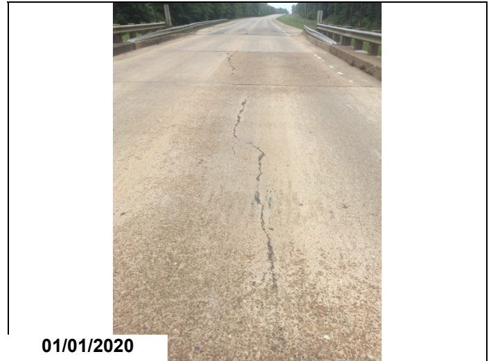
Deck spans 1-2 large unsealed longitudinal cracks up to 1/8" wide.
